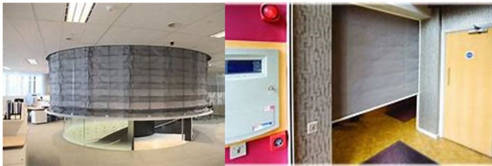
Figure 3: Automatic Fire Barriers
