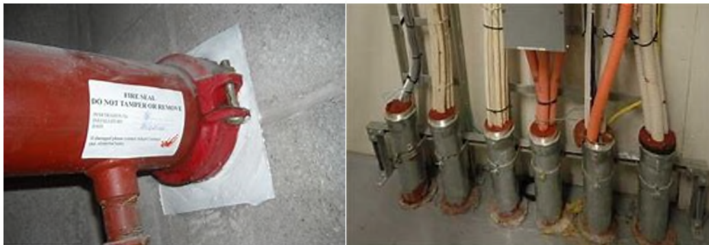
Figure 4: Fire Stopping Through Walls and Floors
